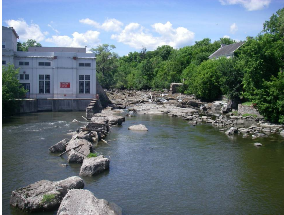
Photo 2 Looking upstream from the Swinging Bridge, July 10, 2009.
