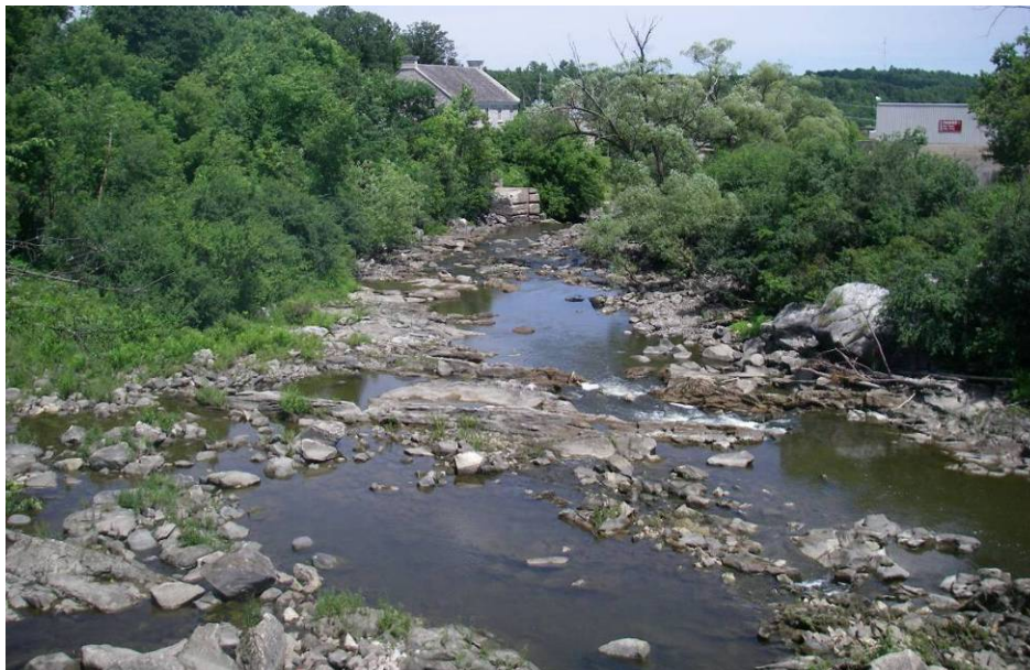
Photo 1 Looking downstream from Dam #1, July 10, 2009.
