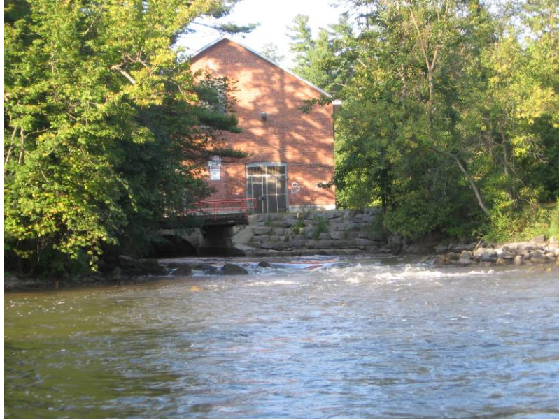
Photo 5 Looking upstream at the tailrace, August 31, 2007.
