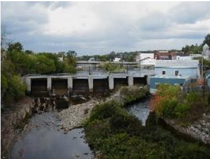
Eganville Dam and Power Station
