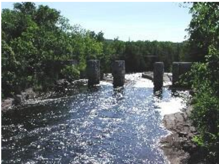
Old Dam Structure at Fourth Chute
